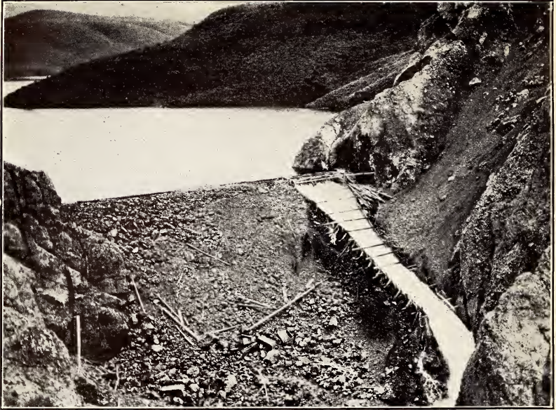
FIG. 1.—EAST CANYON DAM, UTAH, SHOWING TEMPORARY SPILLWAY.
